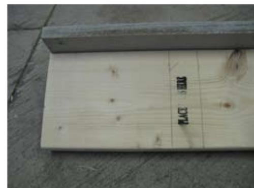
Top plates are marked for trusses as shown.
