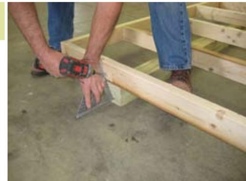
Make sure 2x4 and 4x4's are flush. Secure with 2 1/2" screws on angle as shown.
