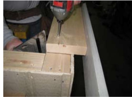
Next install top plate, make sure 2x6 is at the pencil mark as shown on last picture.
