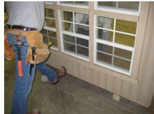
Apply pressure on all walls as shown before securing with 2 1/2" screws.
