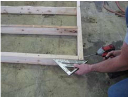
Make sure joist and rim are flush as shown and secure with 2 1/2" screws.
