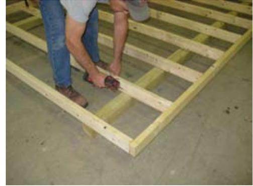
Next measure 16" On Center, and secure 2x4's into 4x4 by toe nailing a 2 1/2" screw on both sides.
