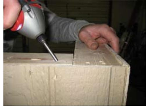
Secure with 2 1/2" Screws on an angle.
