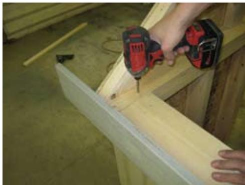
Secure with 2 1/2" screws once gable is in place.
