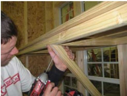
Secure with 2 1/2" screw as shown on top.
