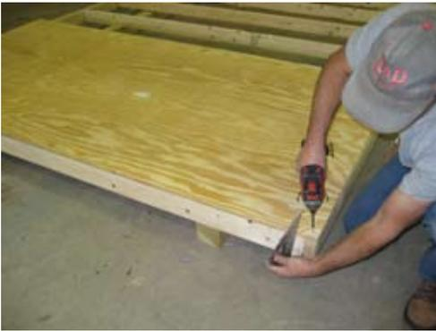
Set sheeting in place using angles to ensure sheeting is flush on both sides. Secure in place by driving 1 1/4" screws through the sheeting and into the 2x4's every 8".
