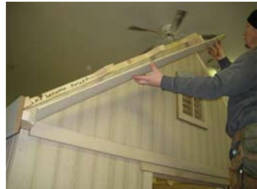
Install 7/16" siding for soffit as shown. Install longer piece first and then shorter one on the other side.
