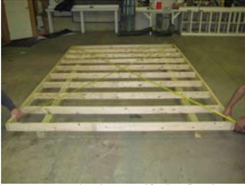
Once 2x4's are in place, verify that flooring structure is square by measuring from corner to corner as shown.
