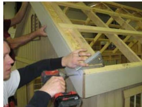
Make sure it is flush on the top of the purlins and secure with 2 1/2" screws.
