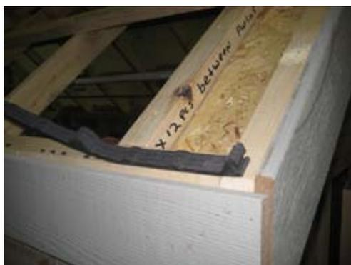
Install rubber closures on bottom edge as shown.
