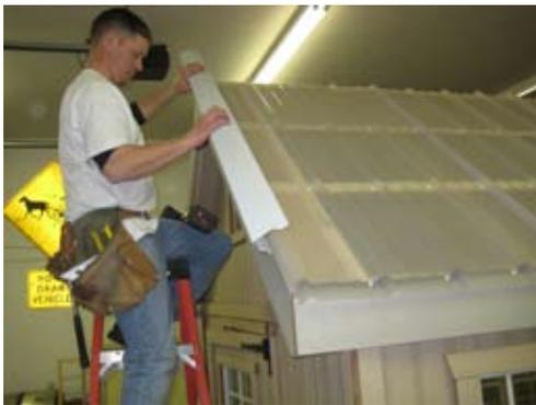
Install rake cover with wider side on top.
