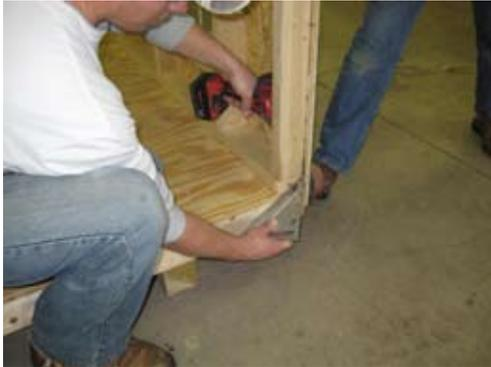
Make sure stud is flush with edge of floor structure using an angle. Apply pressure from outside and secure with 2 1/2" screws.
