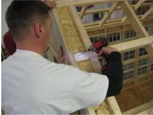
Continue with 2 1/2" screw going from top of purlin into the rake on an angle.
