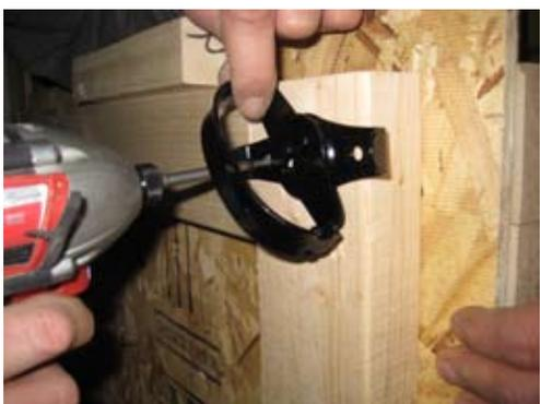
Install inside part and secure with 1 1/4" black head screw.
