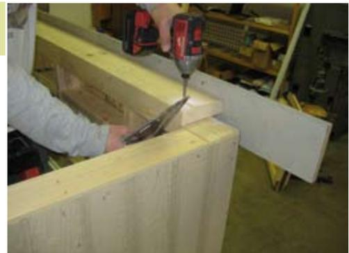
Make sure the Top plate is flush on the inside as well as shown, before fastening.
