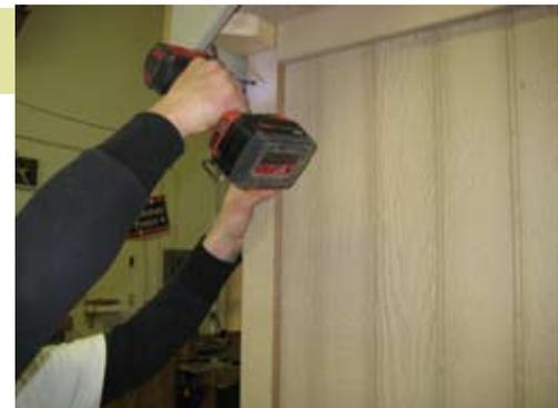
Secure with 1 1/4" screws as needed on all 4 corners.
