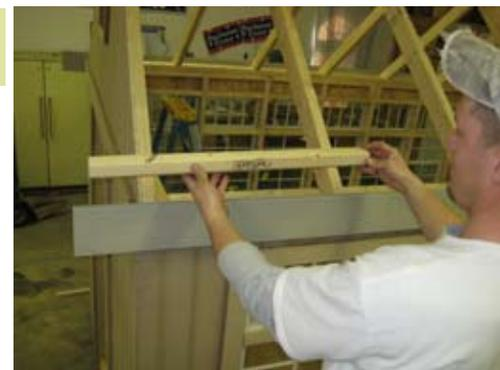
Purlins will be installed on top of trusses for Sunsky to set on.
