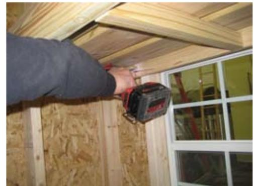
Secure on bottom side with 2 1/2" screw going into 2x4 wall stud.
