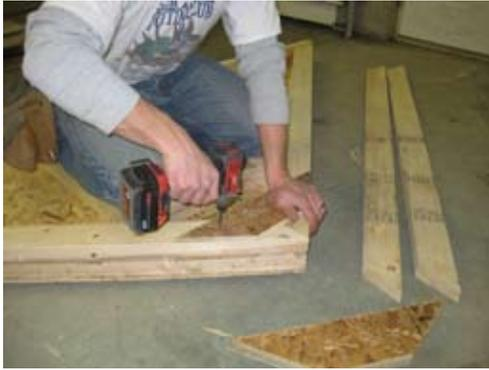
Lay rafters on top of gable so all trusses will be the same. Place Truss gussets as shown and secure with 1 1/4" screws.
