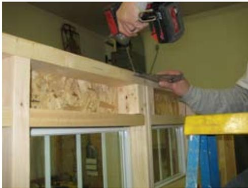
Make sure the walls are flush on the inside and secure with 2 1/2" screws as shown.
