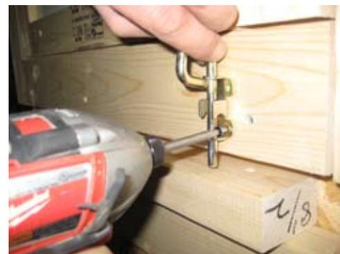
Next install barrel bolt on inside top door and secure with 1 1/4" screw.
