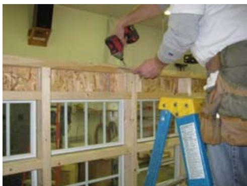
Next make sure walls are flush on inside and secure with 2 1/2" screw.
