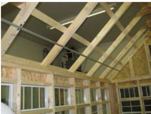
Install C-clamp on every truss.
