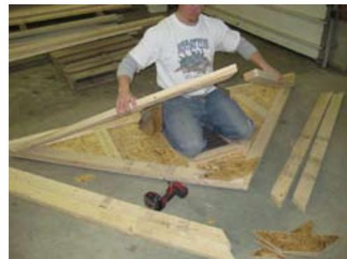
Next locate gable wall and use it for truss assemble as shown.
