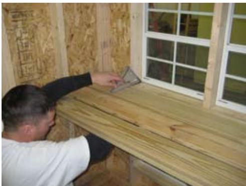
Install first section. Make sure top is flush with window sill.
