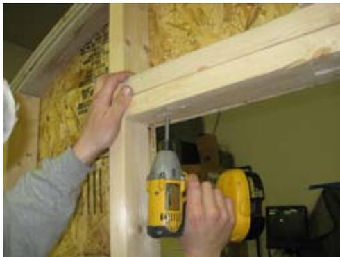
Also insert 2 1/2" screw from bottom of header up into 2x4 as shown.
