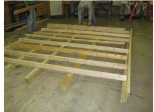
Next layout 2x4's for floor joist.
