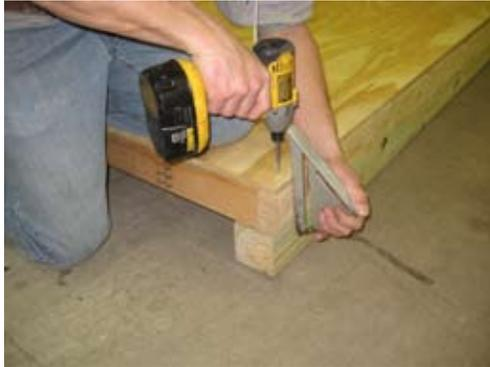
Start at corner as shown. Use square to make sure plywood is flush and secure with 1 1/4" screws as shown.
