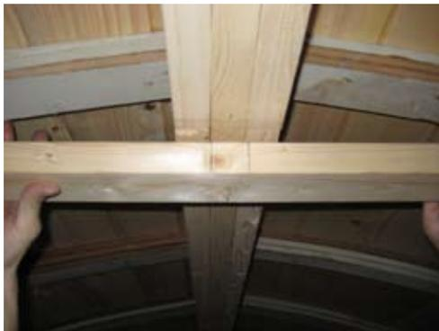
Locate the center mark on collar tie and make sure it center with 2x6 as shown. Secure with 2 1/2" screws at center and each end.
