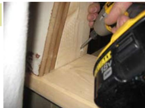
One screw on outside and one on each side of truss as shown.
