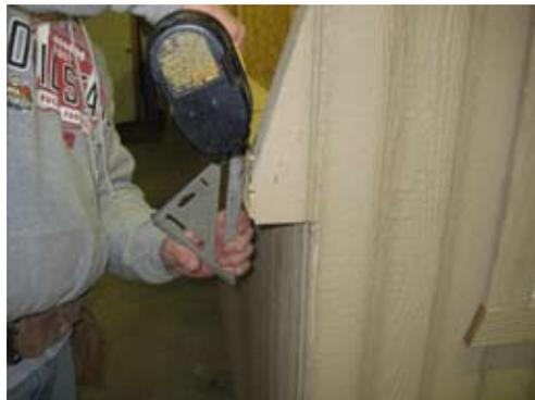
Make sure all four corners are flush on outside of top plate as shown.
