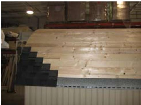
Install shingles as shown and secure with 3/4" nails.
