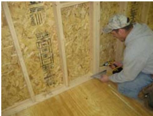
Insert 3 to 4 2 1/2" screws, where 2x4's meet to tie wall together.
