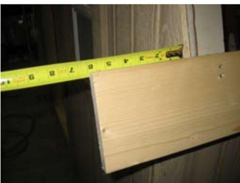
Start with short piece. 1x6 needs to overhang 6" from siding. Secure with 2 1/2" screws.
