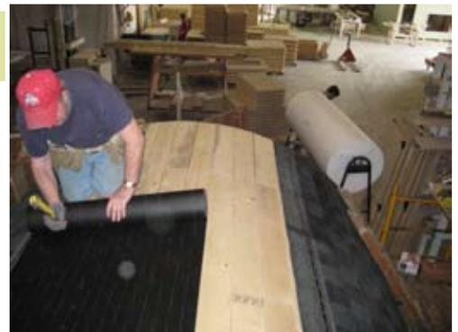
After both sides are 3/4 ways up as shown. Roll out felt paper as shown.
