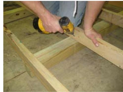
After floor is squared up secure joist in center rows with 2 1/2" screws 1 on each side.
