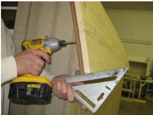
Use square to make sure rafter trim is flush on bottom as shown. Secure with 1 1/4" screws.
