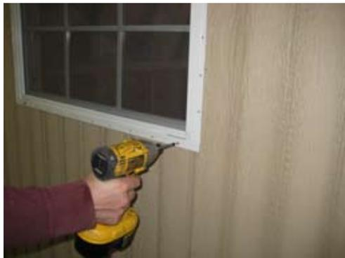
Make sure window is centered in opening and secure with 1 1/4" screws as needed.
