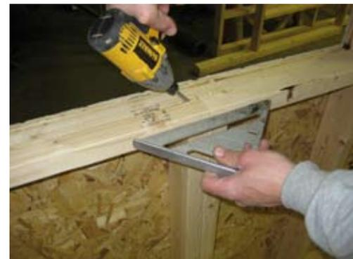
This is where the window opening meets. Make sure plates are flush, secure with 2 1/2" screws.
