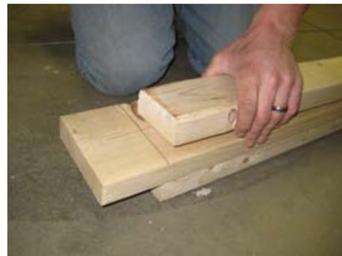
Next flip 2x6 over and install 2x4 on bottom side as shown.
