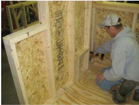
While applying pressure on outside, secure wall with 2 1/2" screws.
