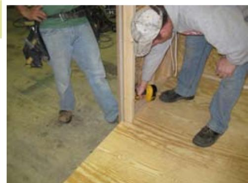
Apply pressure on the outside as shown and secure with 2 1/2" screws.
