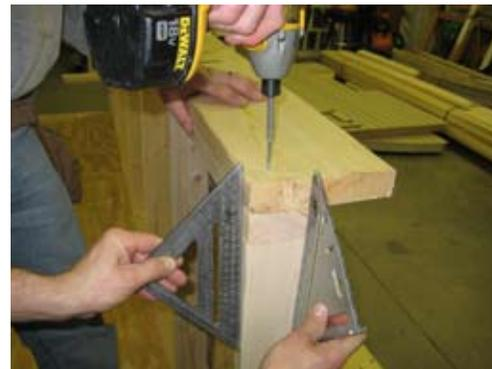
Next install top plates. Make sure plates are flush on inside and at end as shown. Secure with 2 1/2" screws.
