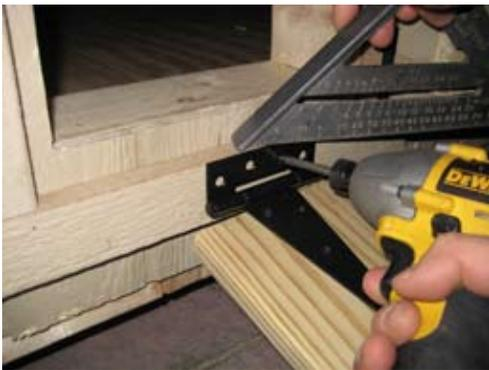
Keep hinge flush on top of trim as shown and secure with 1 1/4" screws.
