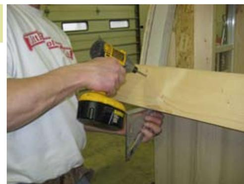
Make sure bottom of 1x6 is flush with 2x8 Top Plate as shown.
