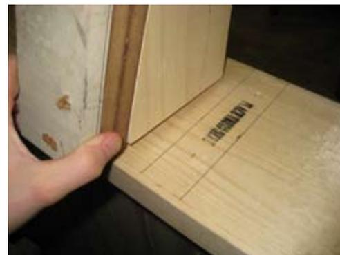
2x8 Top Plate is marked where to install truss.
