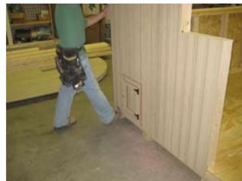
Position wall in place and apply pressure on outside as shown.
