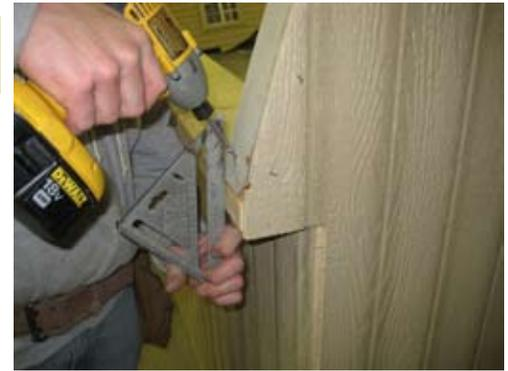
Make sure rafter is flush with 2x6 top plate and secure with 2 1/2" screws.
