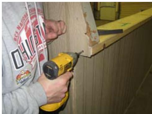
Insert 1 1/4" screw through siding into 2x6 Top Plate.
