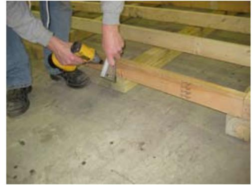
Next make sure 4x4's are positioned in place and secure with 2 1/2" screws as shown.
