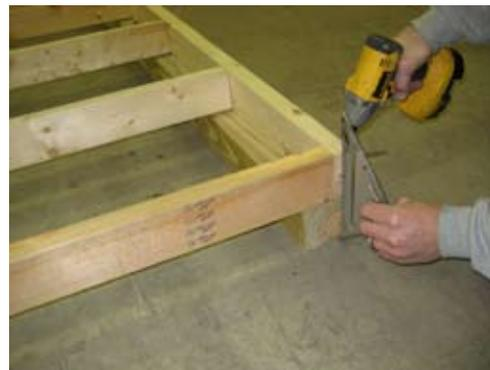
Next make sure 4x4 is flush with rim as shown and secure with 2 1/2" screws.
