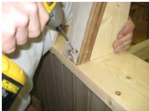
Once truss is in position secure with 2 1/2" screws.
