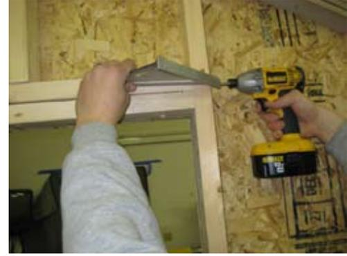
Use square to make sure 2x's are flush as shown and secure with 2 1/2" screw.
