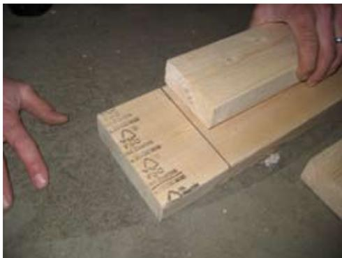
Lay out 2x6 and screw 2x4 on top. Stay even with pencil mark.
