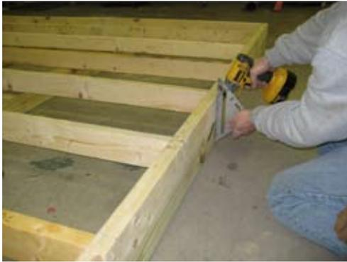
Continue all the way out around as shown so 2x4 is flush with 4x4 and secure with 2 1/2" screws.
