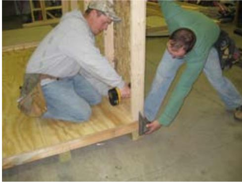
Set wall up and apply pressure on outside as shown. Also make sure wall is flush on end as shown. Secure with 2 1/2" screws.
