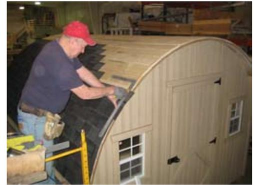
Make sure shingles are cut off at 1/2" over the edge of the roof.
