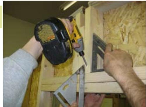
Secure all loose 2x4's with 2 1/2" screws as shown.
