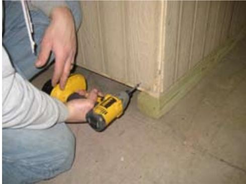
Next secure the bottom edge all the way around with 1 1/4" screws 8" on center.
