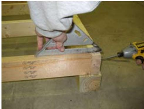
Use square to make sure joist is flush on top of rim as shown and secure with 2 1/2" screws.
