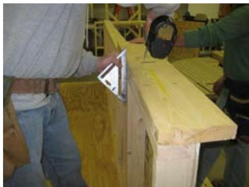
Continue with top plates and make sure it is flush on inside as shown.
